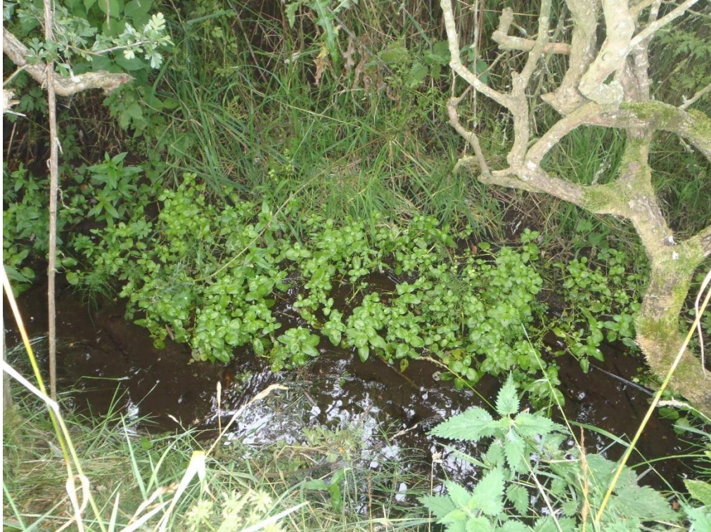
Picture 5: showing the ditch on the eastern boundary
